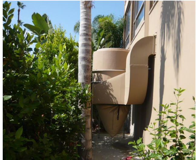
OPL-300 Filter – Installed Outdoors Keeps Environment Free of Dryer Lint
